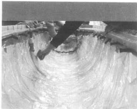
Figure 8. Final Lay-up After Vacuum Bagging.
